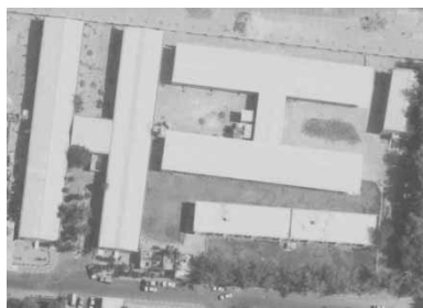
Figure 5. The architectural design of Al Ain Hospital reflecting its symbol (H). Note the 'H' shapes on the aerial photograph of 1984. The figure shows how non-spatial characteristics (design intention) can be deduced from remote sensing.
